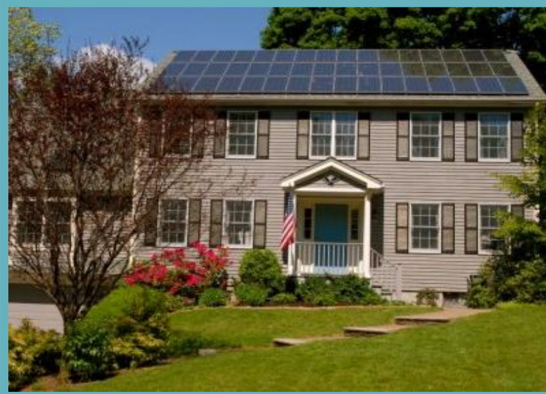
Solar Photovoltaic (PV)
