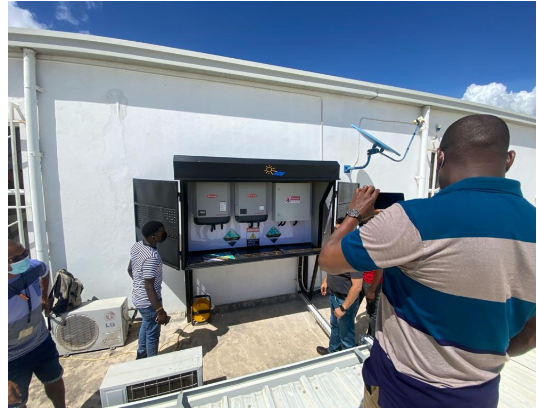
DHL -Dar es salaam-Grid tie PV System 36.72kWp =68 @ 540Watts
