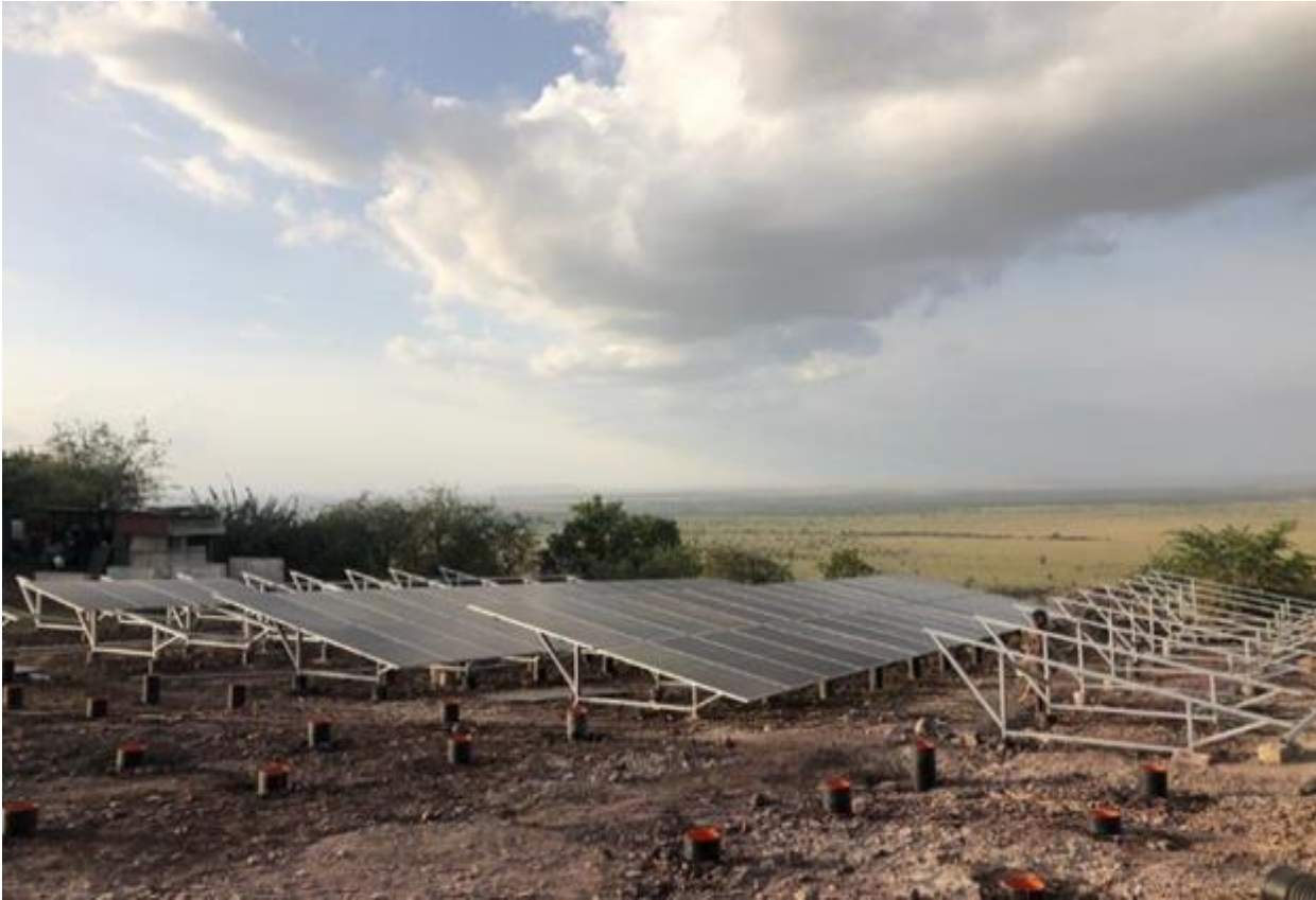
Kimarishe Lodge/Serengeti National park –Offgrid PV System (Ground mount) 243kWp =450@ 540Watts
