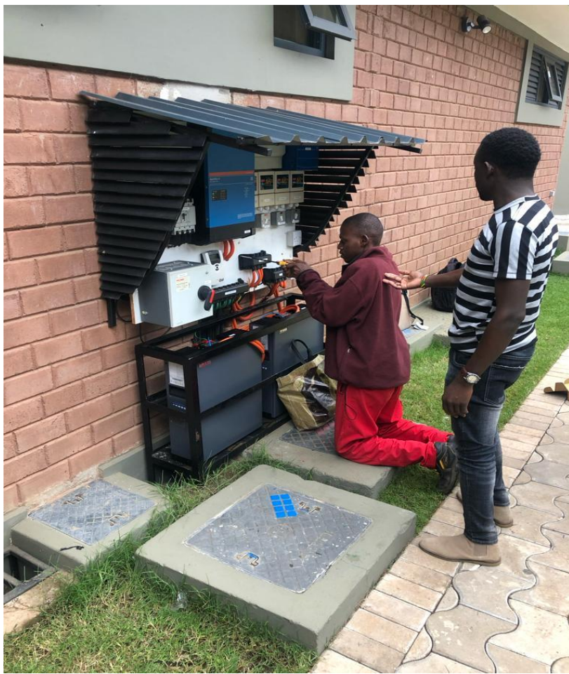
Backup system only tied to a battery bank & grid (no solar panel)
