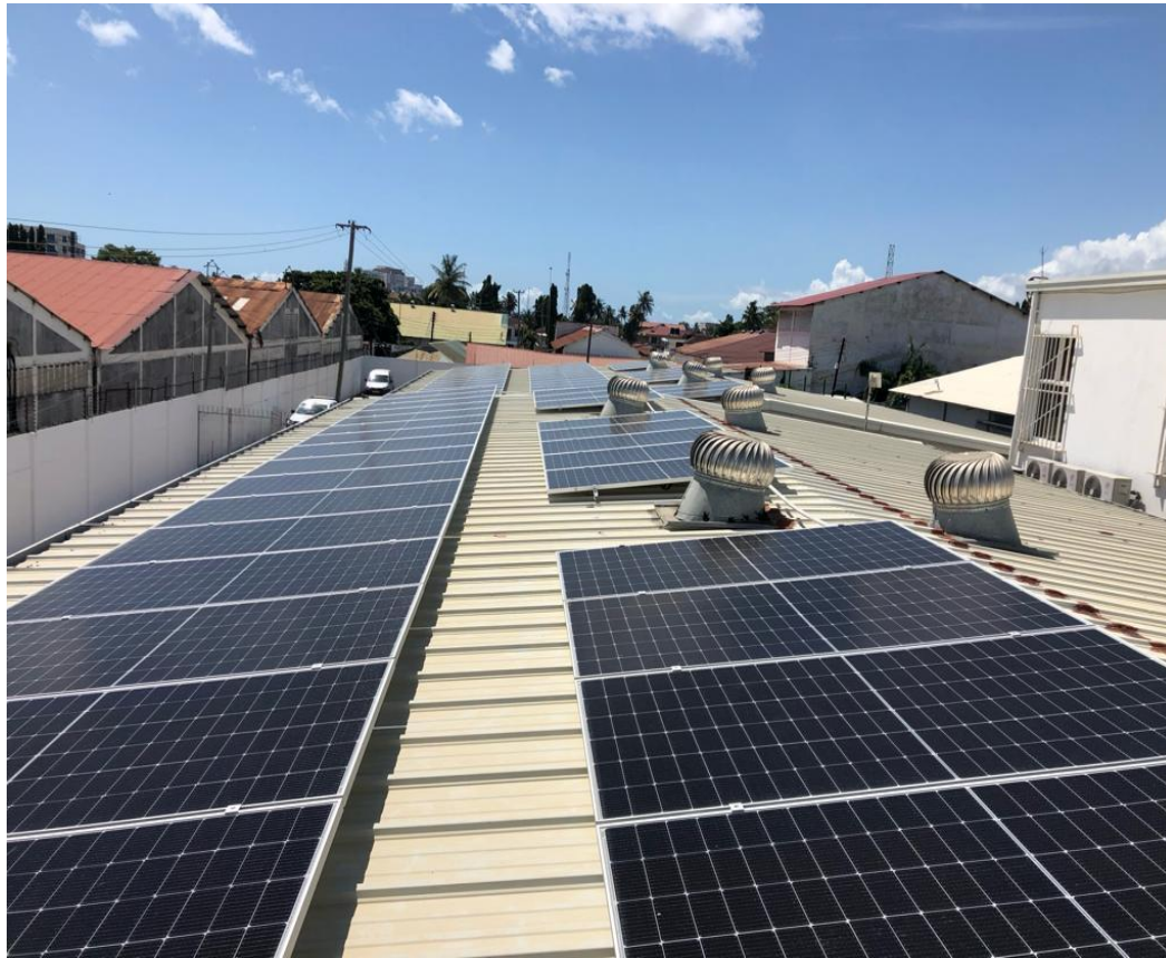
DHL -Dar es salaam-Grid tie PV System 36.72kWp =68 @ 540Watts
